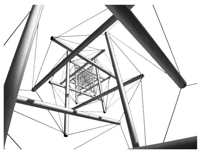
Tensegrity is a synthesis of the names 'tensional' and 'integrity'. It is based on "*teamwork*" of tension and compression forces. Although the image may look confusing, these structures are very simple. All you need are some poles, some cable, and good engineering. This results in a beautiful 'tensegrity-tower' where the poles almost float in the air; as shown above
